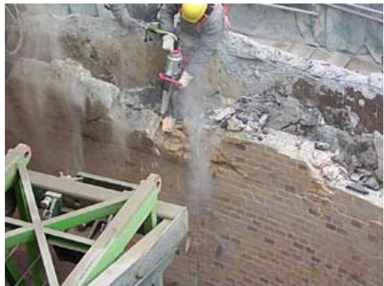
For the demolition of an industrial chimney the inner wall was systematically dismantled using a LUKAS spreader. The demolition of the chimney could not be completed using conventional methods as a blast at this location was not possible.
